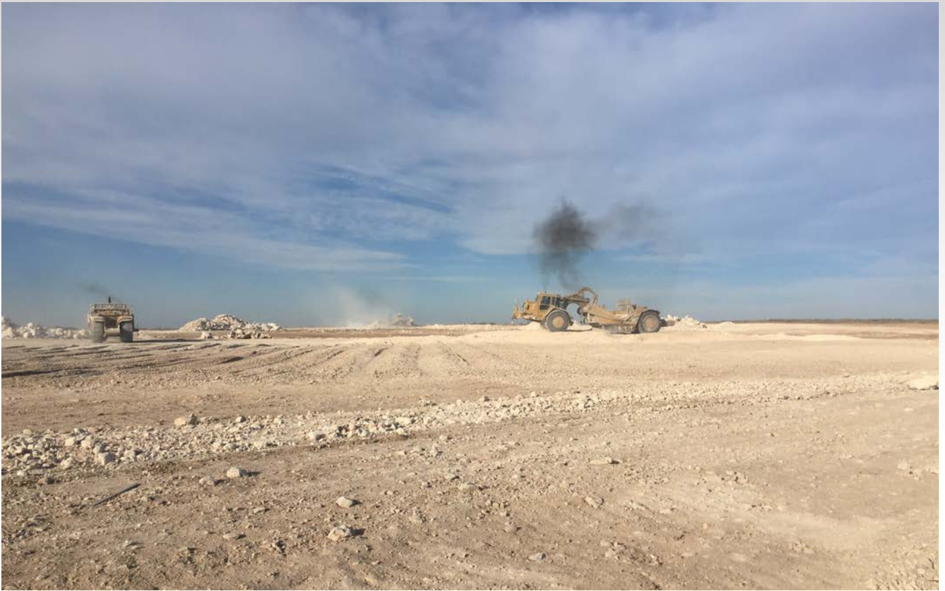
Pictured above: K5 Services oilfield pad construction in west Texas.
