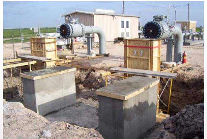
Separator Foundation Slab & Piers
